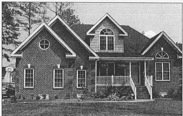
Elevated home on crawl space foundation
