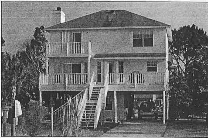
Elevated home on pile foundation
