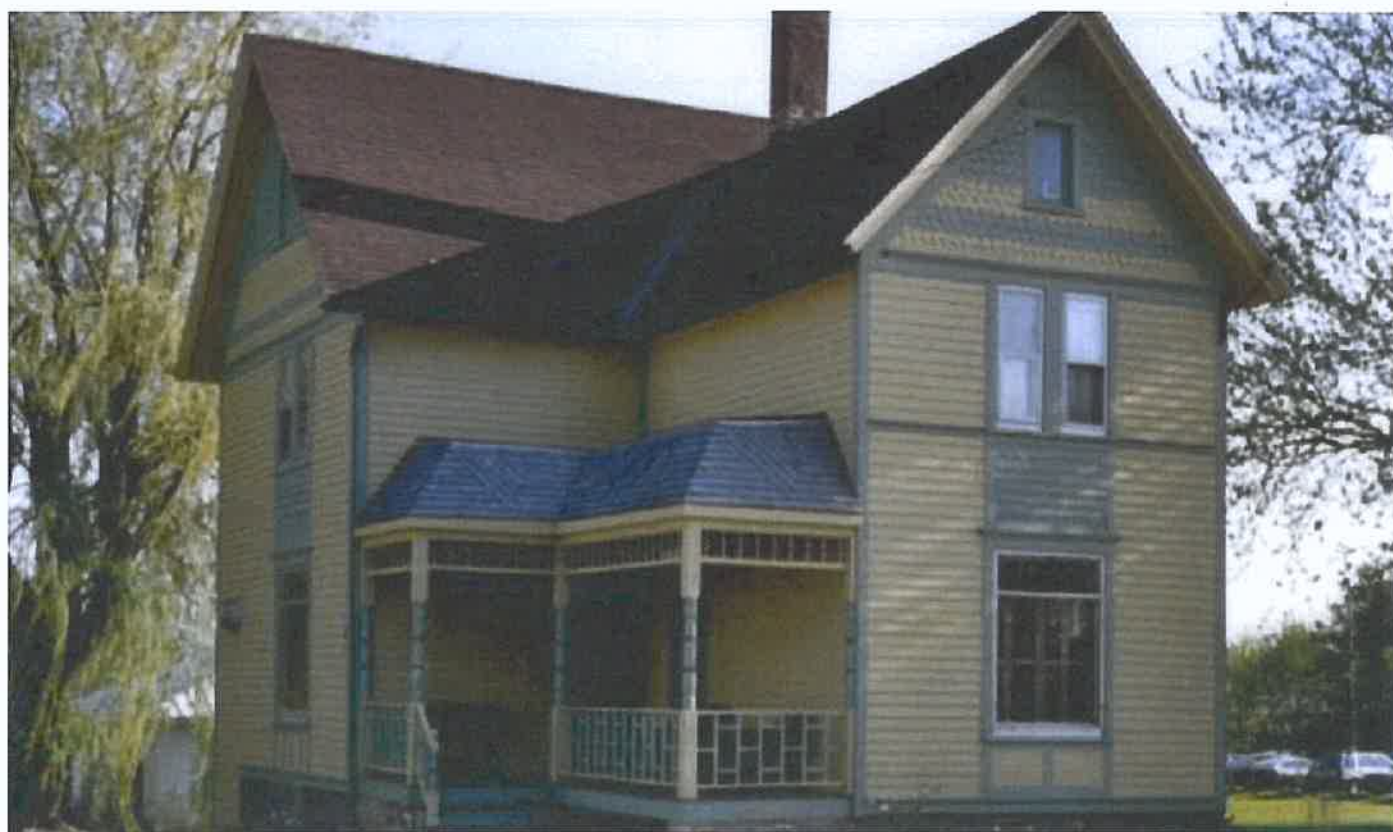
2011 - After the renovation
