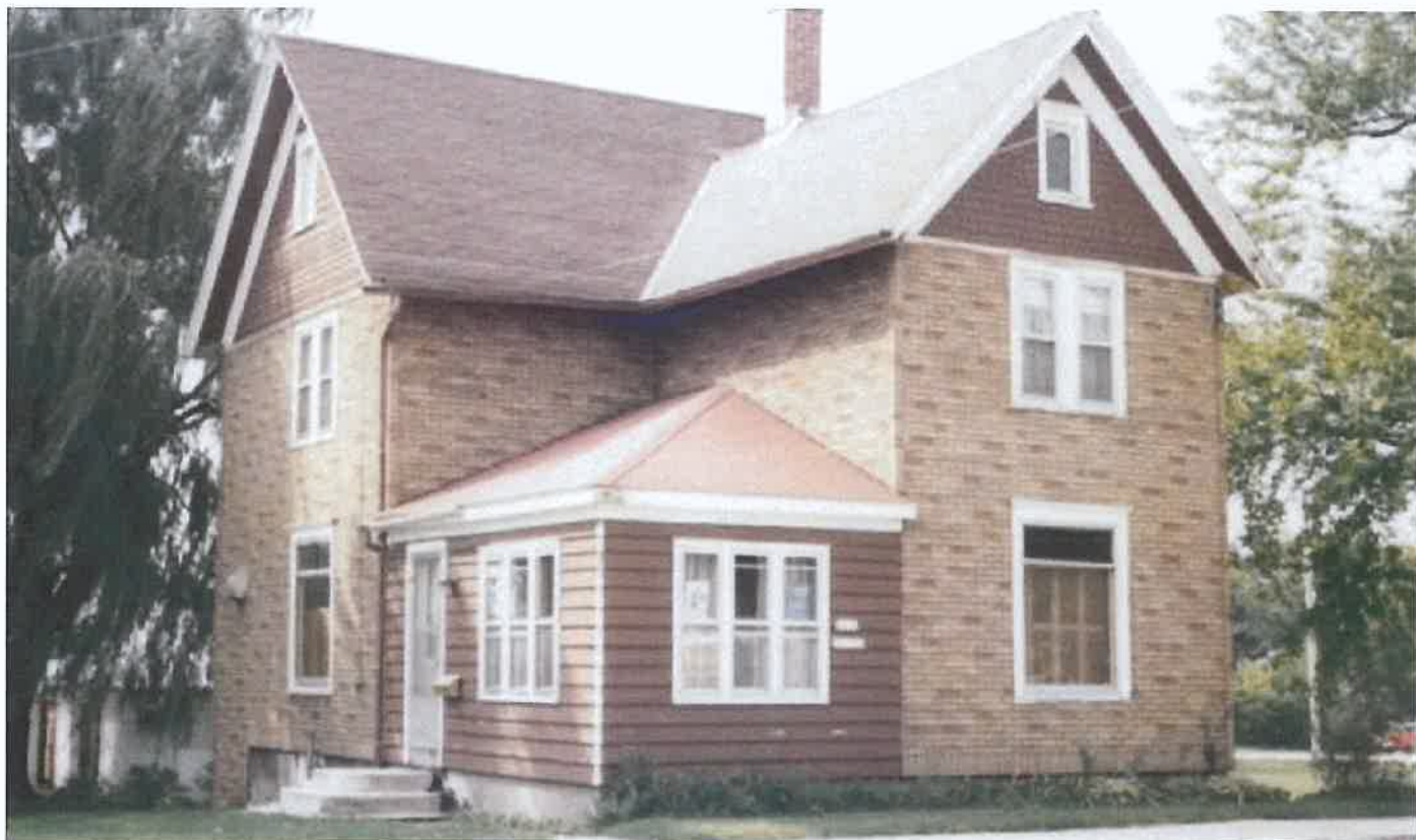
1983 - Before the renovation.
