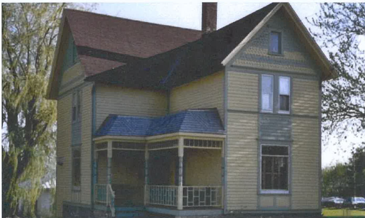
2011 - After the renovation
