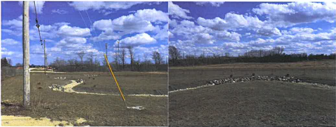
Looking east to wetland area (post WIDOT project)
