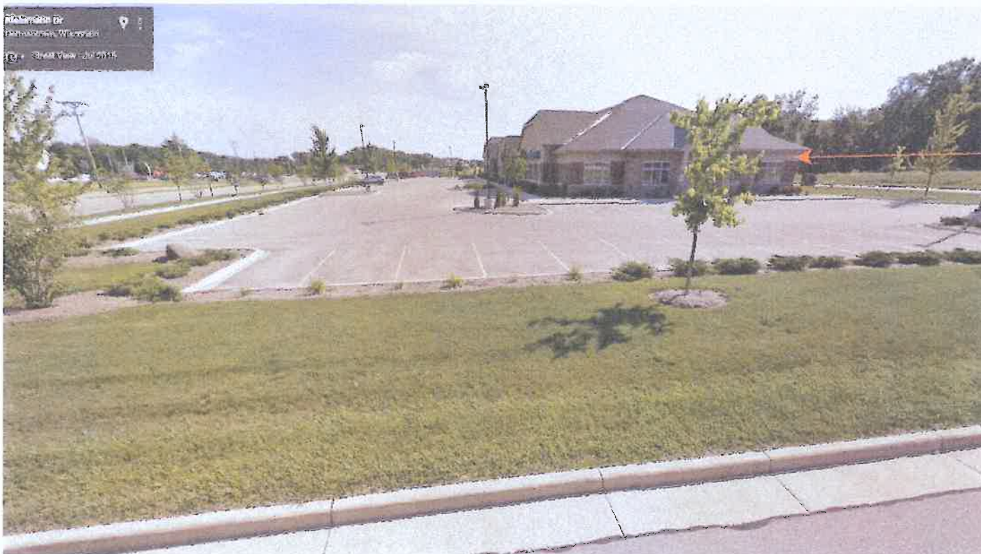
Sign Location on North Elevation
