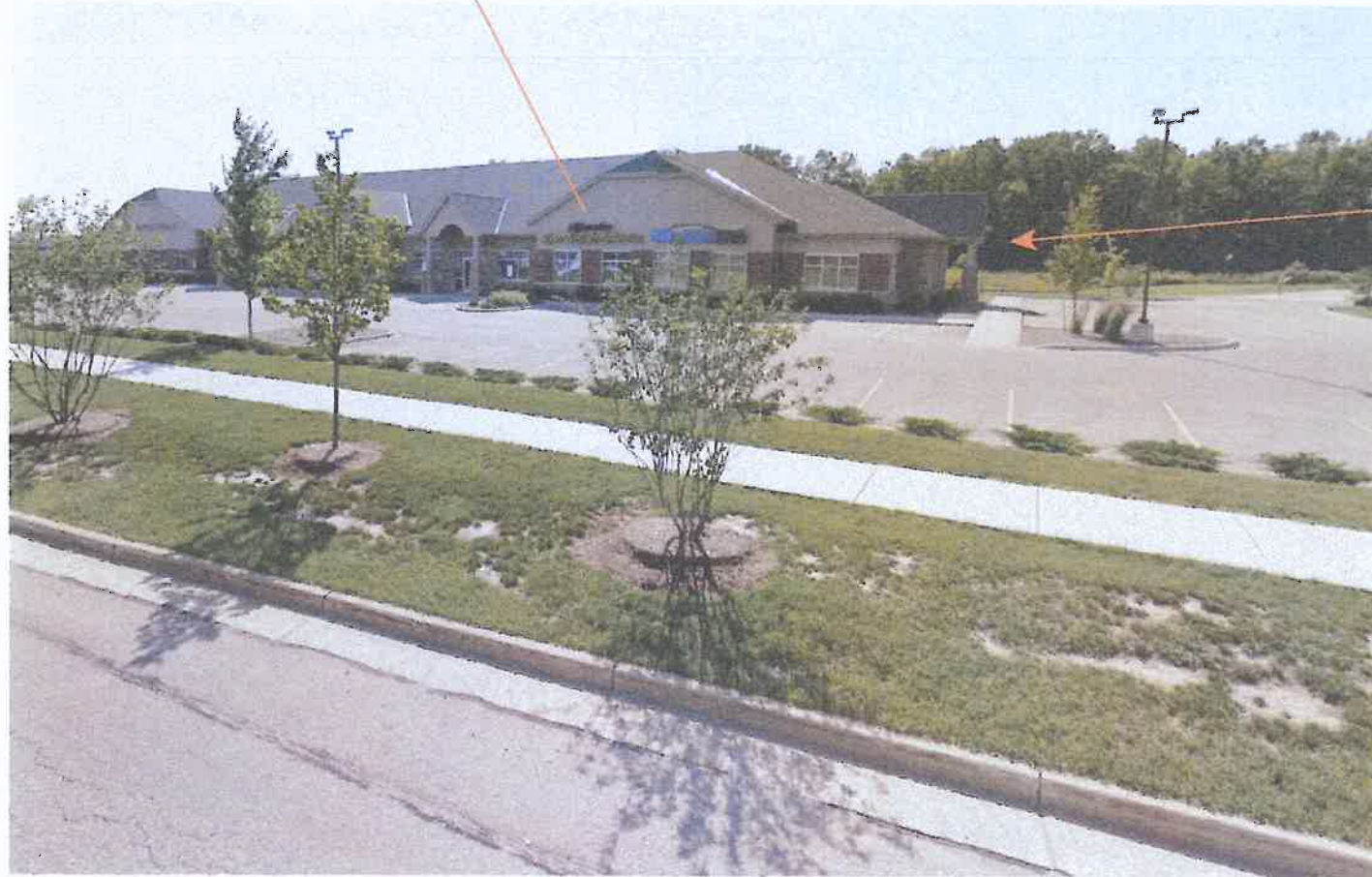
East Elevation, other tenants
