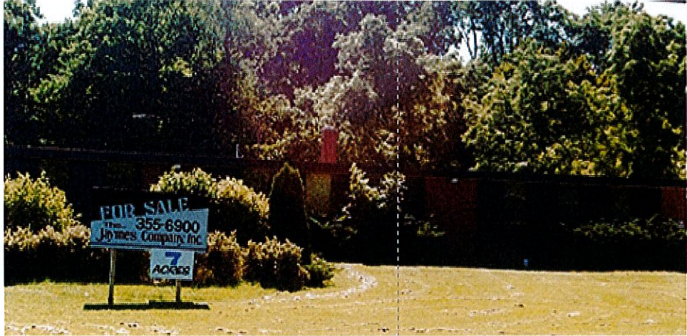
FRONT OF BUILDING AFTER RENOVATION
