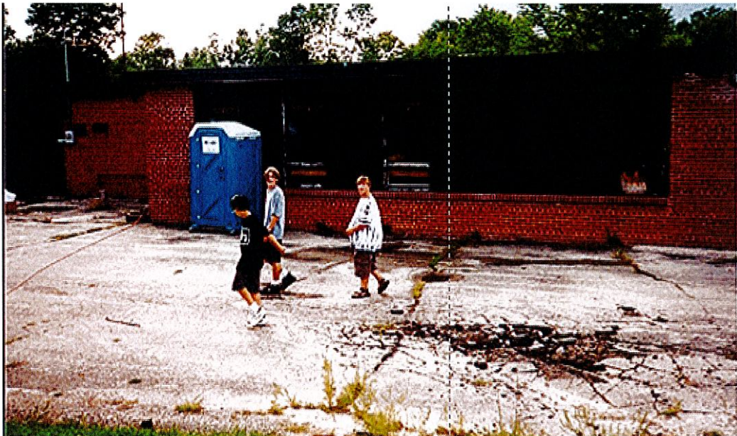
BACK OF BUILDING WHEN PURCHASED BY ADVANTAGE RESEARCH
