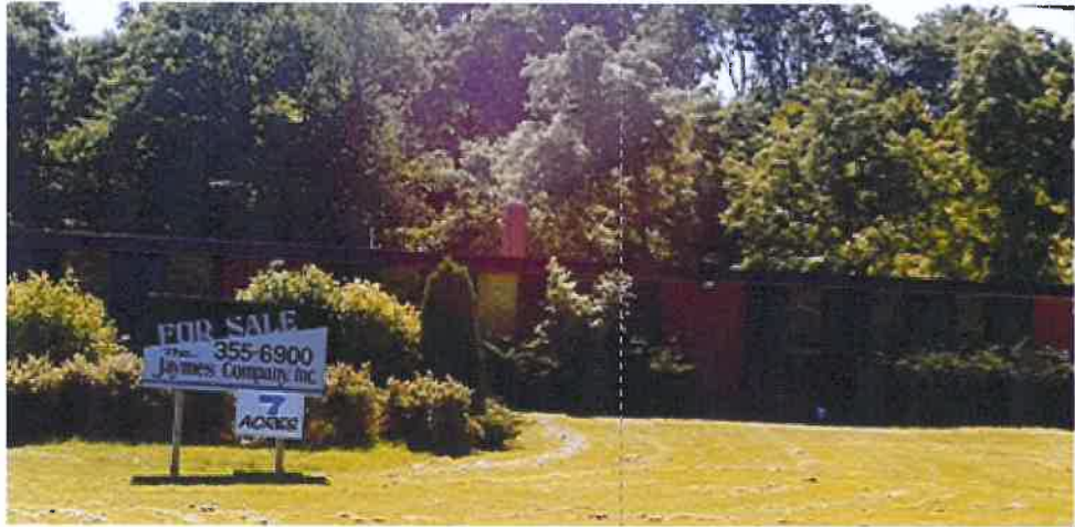
FRONT OF BUILDING AFTER RENOVATION
