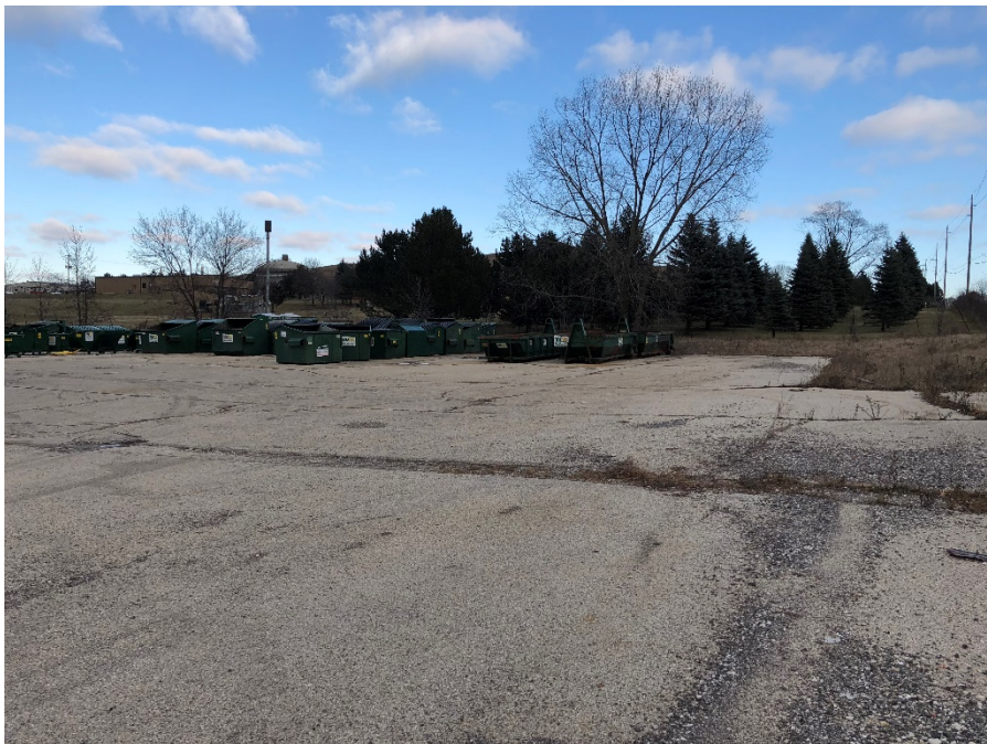
Existing lot at Port-o-let facility. (Dec. 2018)
