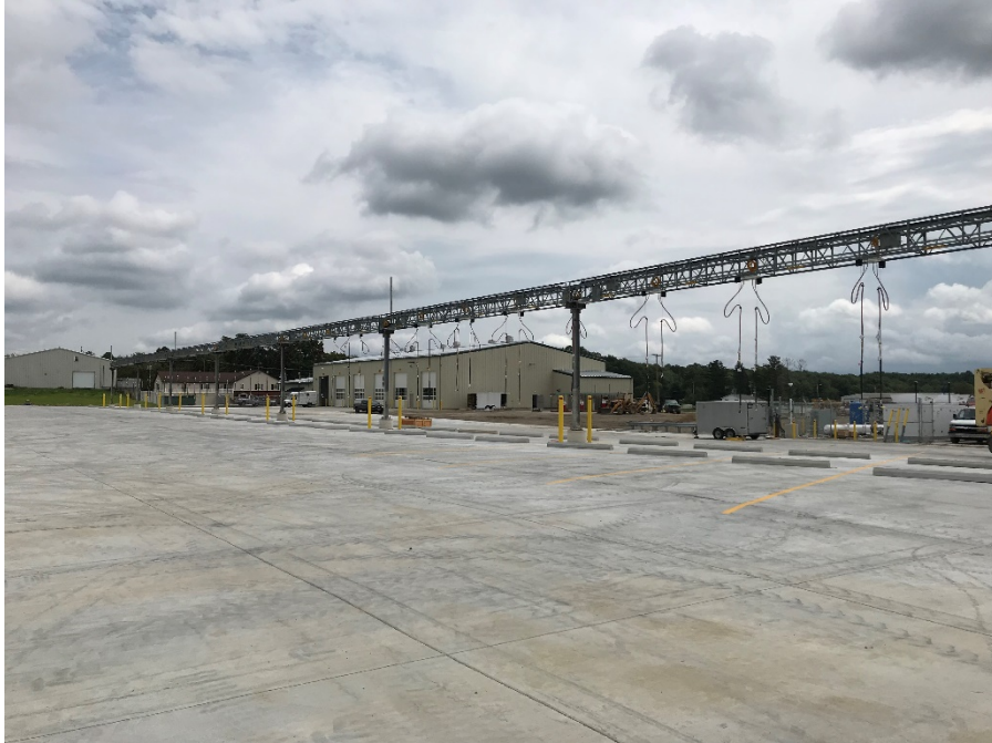
CNG fueling area.
