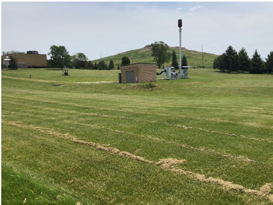
Existing burn-off flare and maintenance building. (July 2018)
