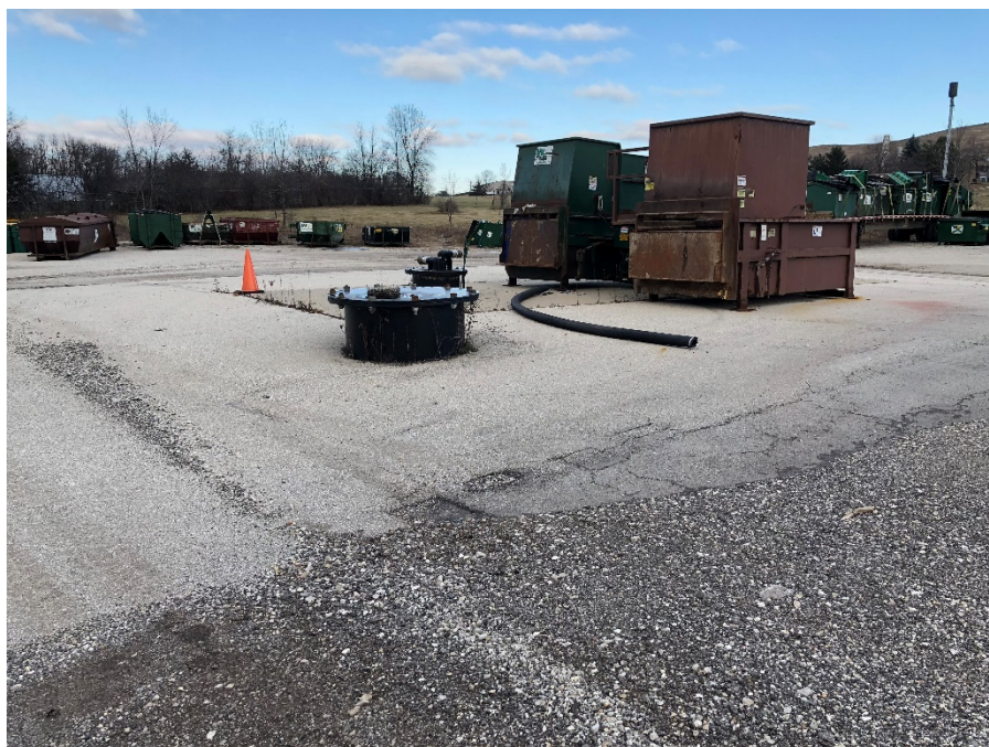
Abandoned underground storage tank. (Dec. 2018)
