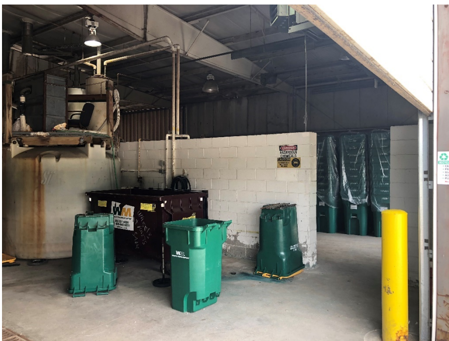
Interior of WM Port-o-let maintenance building. (July 2018)
