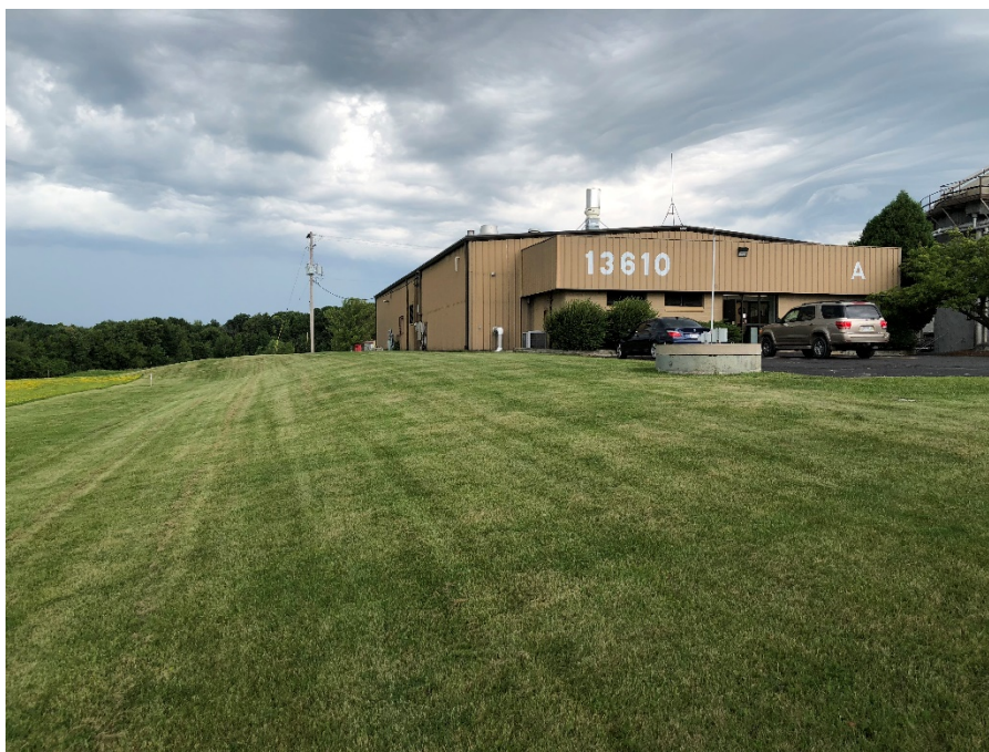
Leachate management facility. (July 2018)
