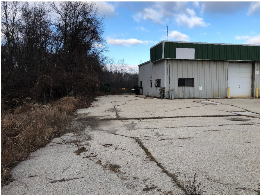
Existing asphalt lot.
