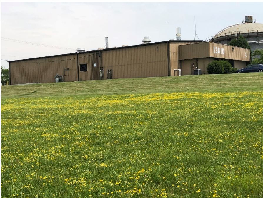
Existing leachate management facility. (July 2018)
