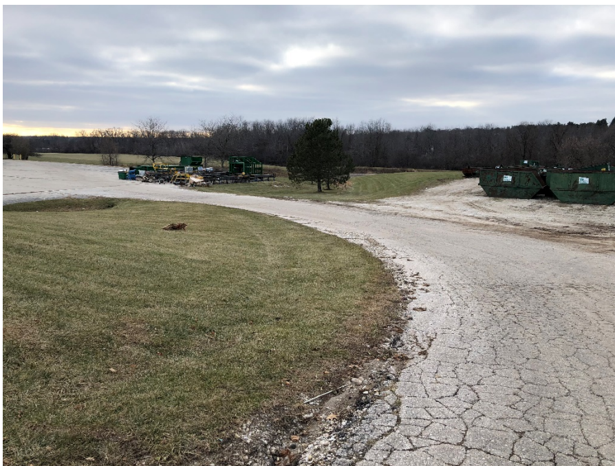
Existing asphalt drive. View facing southwest. (Dec. 2018)
