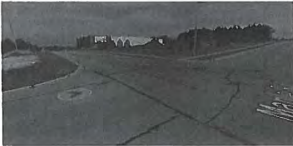
Maple Rd SB view looking EB on Freistadt Rd
