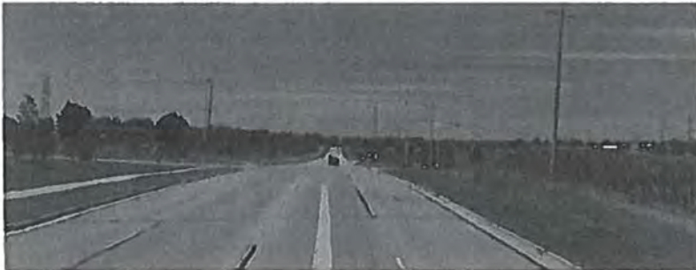
Freistadt Rd WB view looking at Maple Rd (2016 - before exclusive lanes striped)
