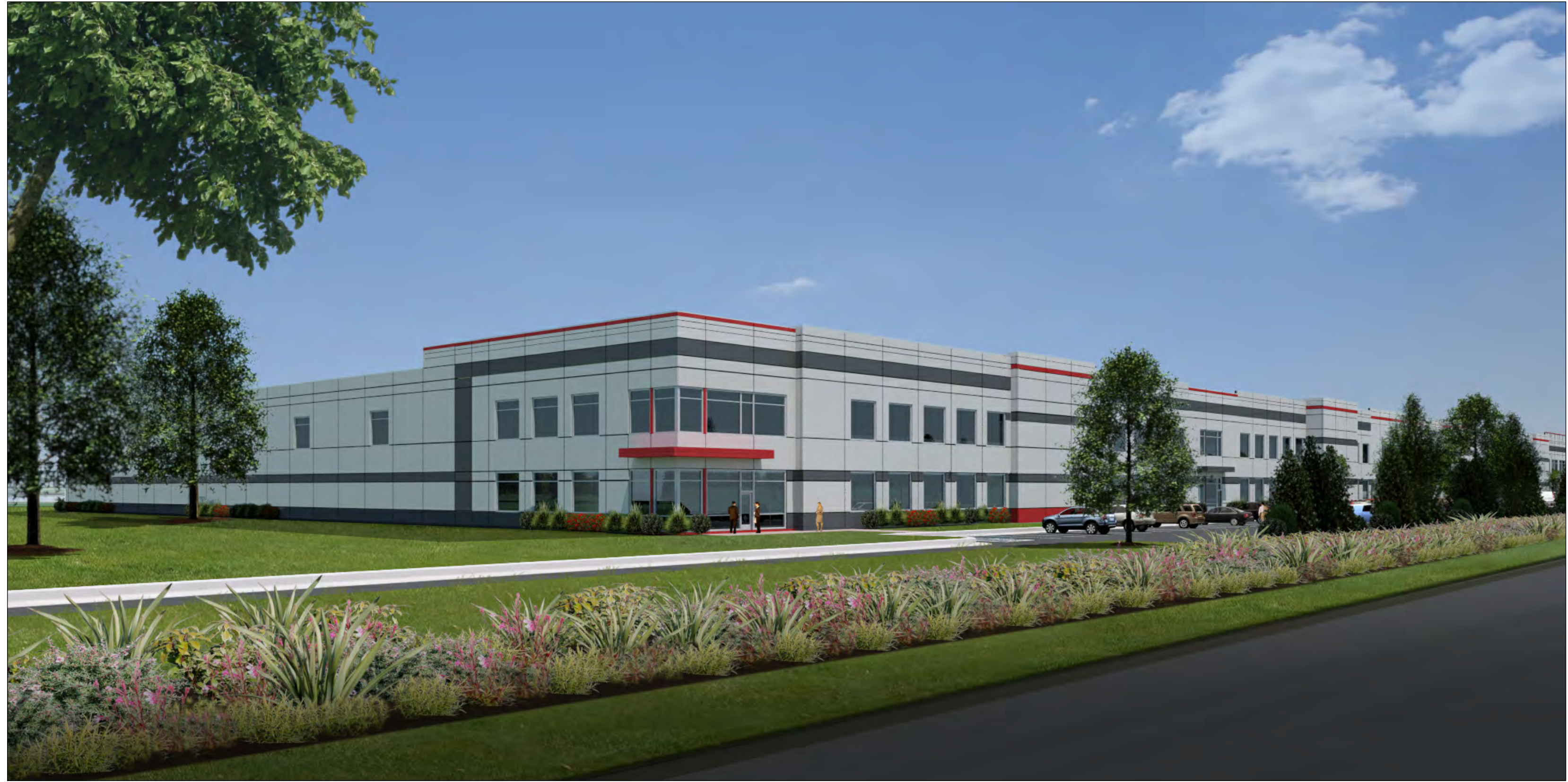
2 NORTH BUILDING - VIEW OF NORTH EAST CORNER LOOKING SOUTH WEST NO SCALE
