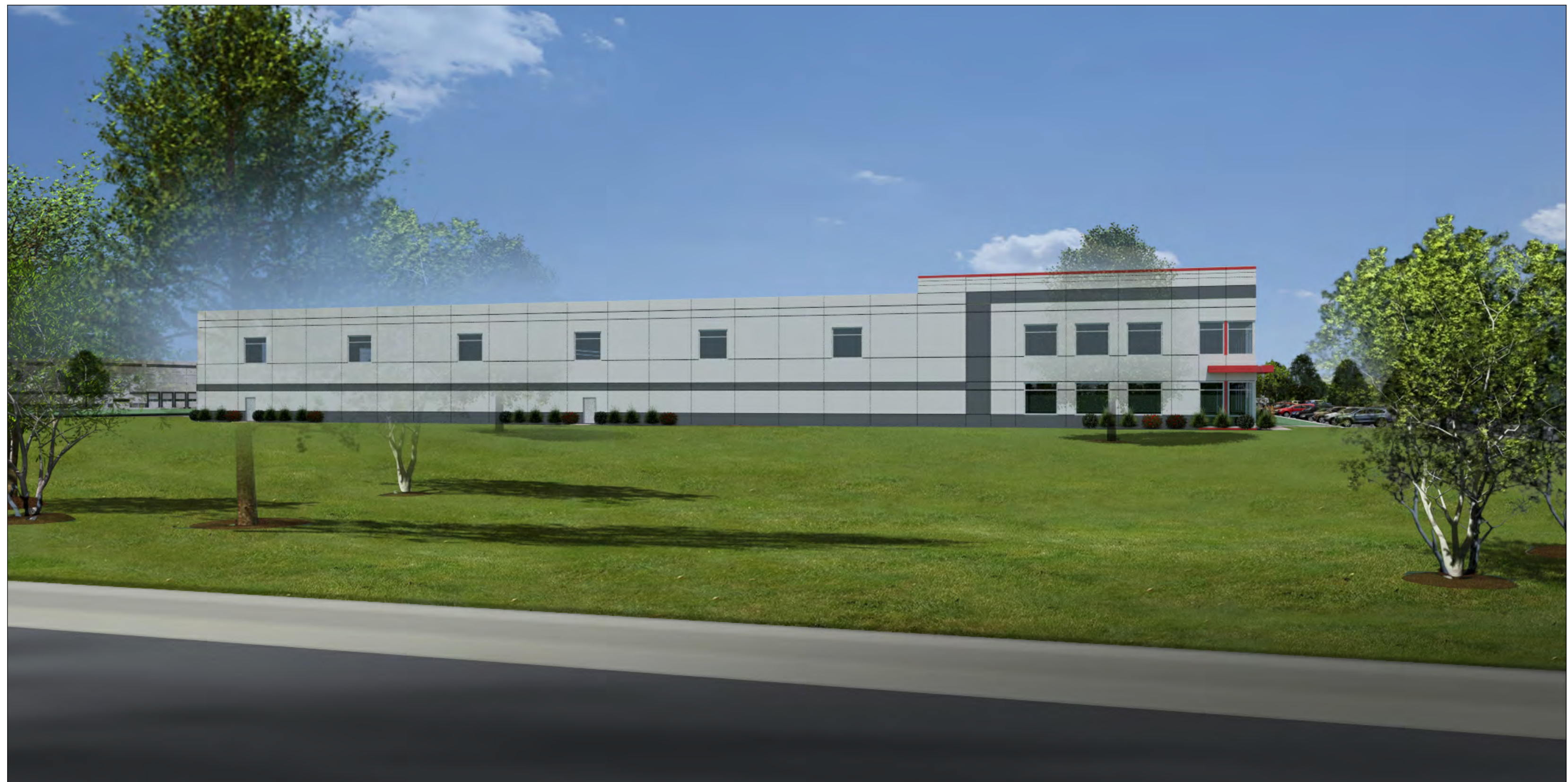
4 NORTH BUILDING - VIEW OF EAST WALL LOOKING WEST NO SCALE
