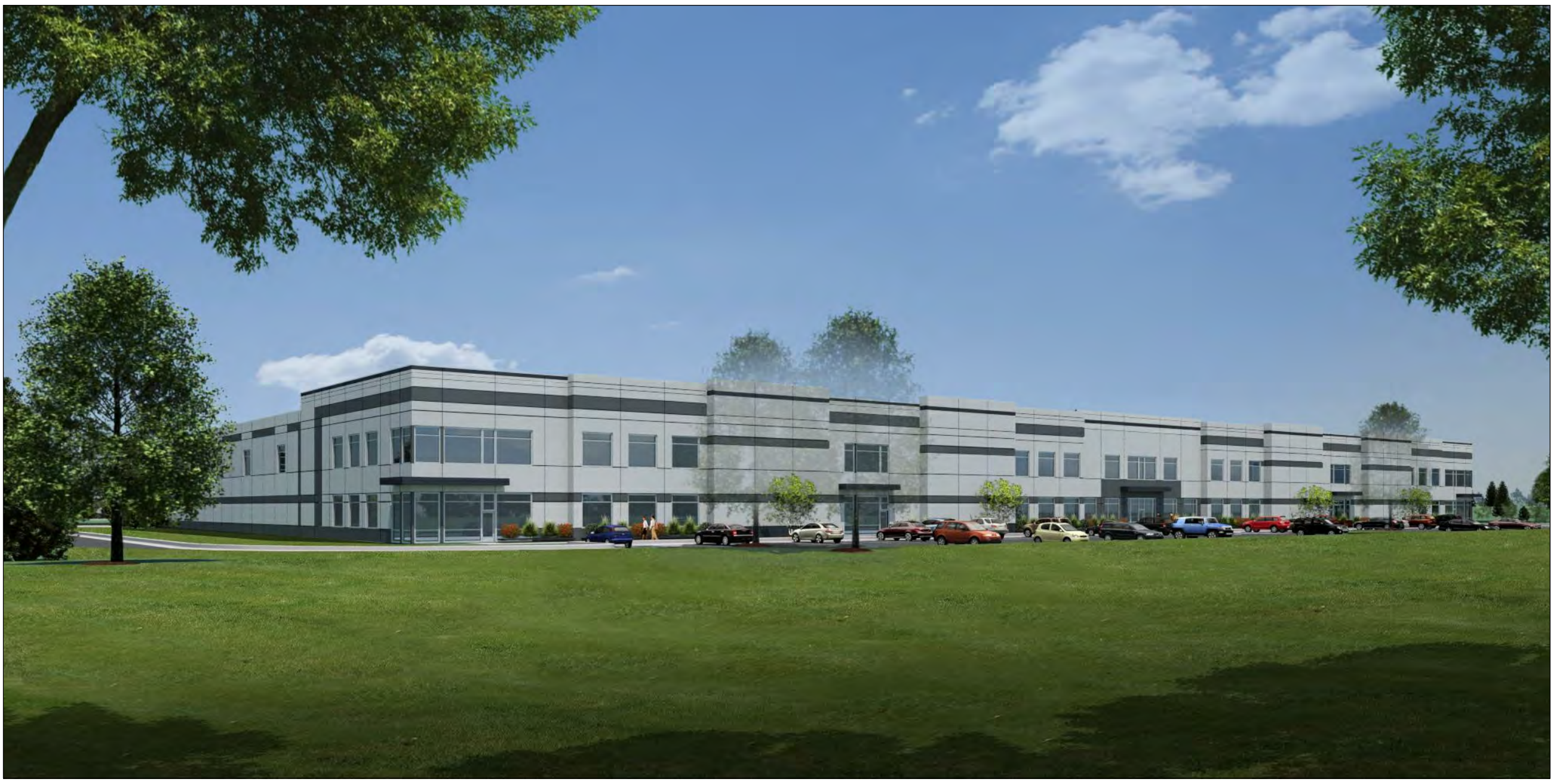
4 SOUTH BUILDING - VIEW OF SOUTH WEST CORNER LOOKING NORTH EAST NO SCALE
