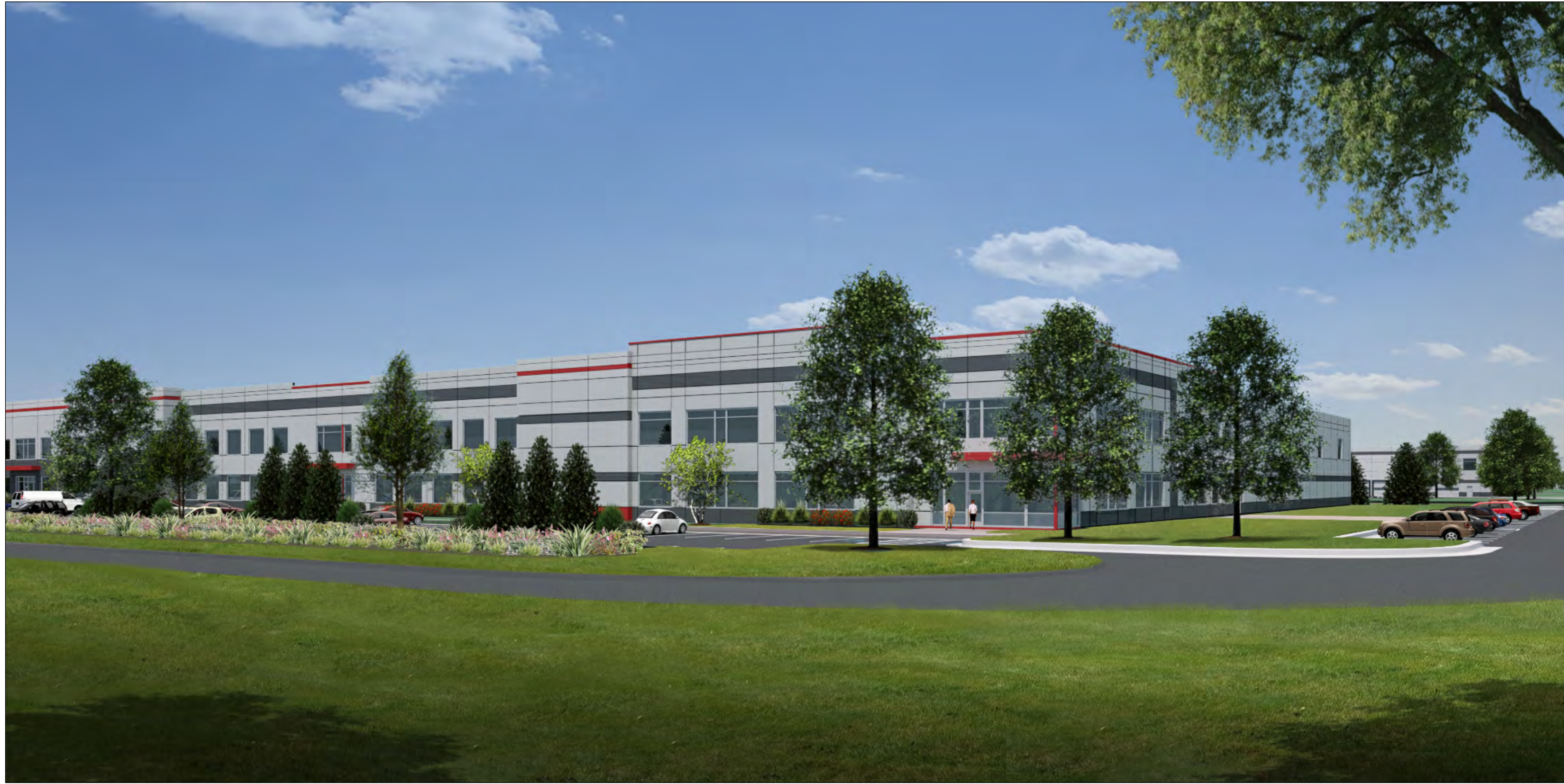
1 NORTH BUILDING - VIEW OF NORTH WEST CORNER LOOKING SOUTH / SOUTH EAST NO SCALE
