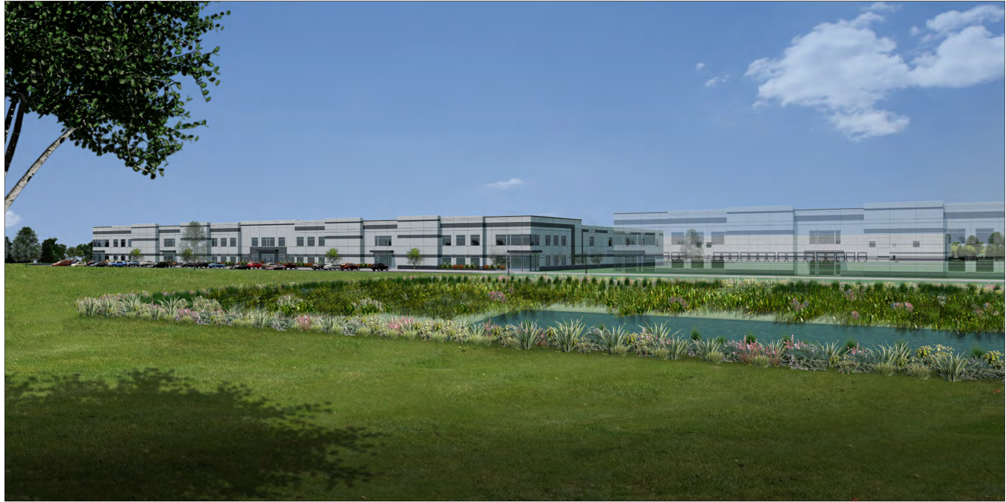
2 SOUTH BUILDING - VIEW OF SOUTH WALL LOOKING NORTH / NORTH WEST NO SCALE
