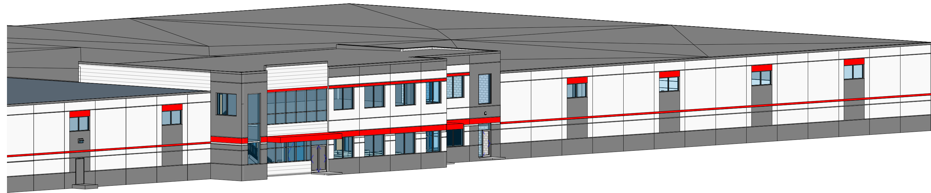
10 NW VIEW OF ENTRANCE
