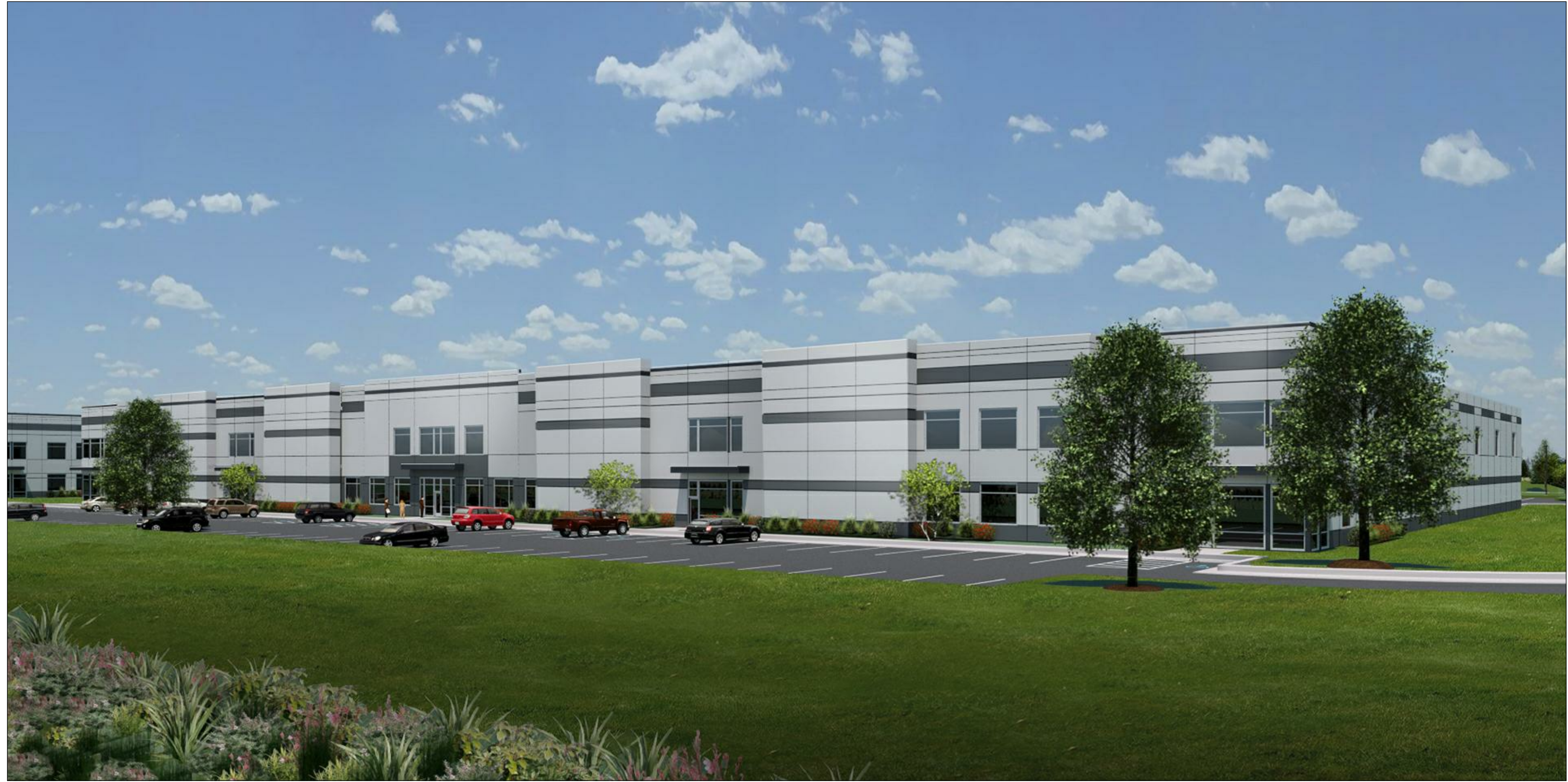
2 SOUTH EAST BUILDING - VIEW OF SOUTH EAST CORNER LOOKING NORTH / NORTH WEST NO SCALE
