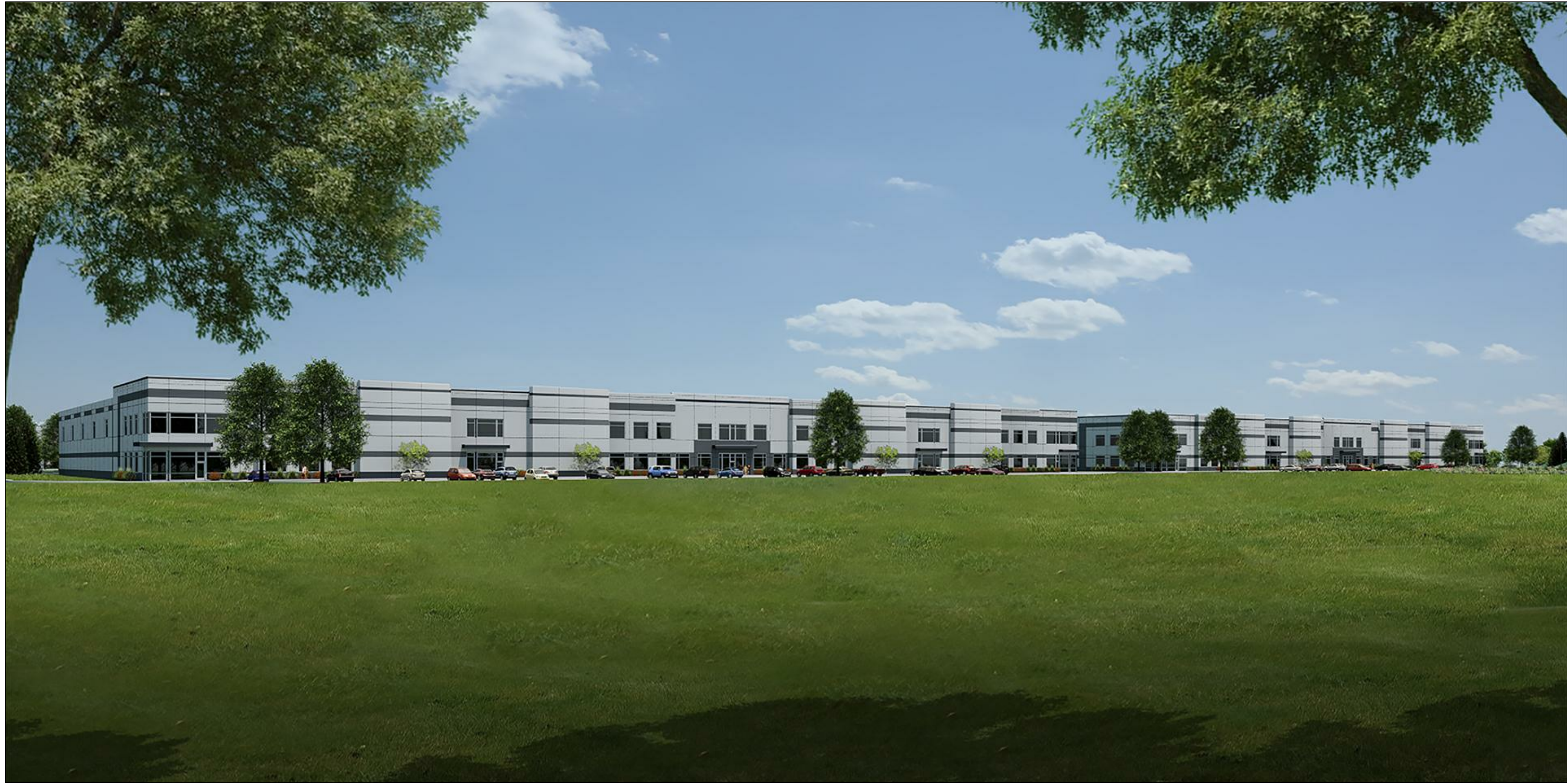
1 SOUTH WEST BUILDING - VIEW OF SOUTH WEST CORNER LOOKING NORTH / NORTH EAST NO SCALE
