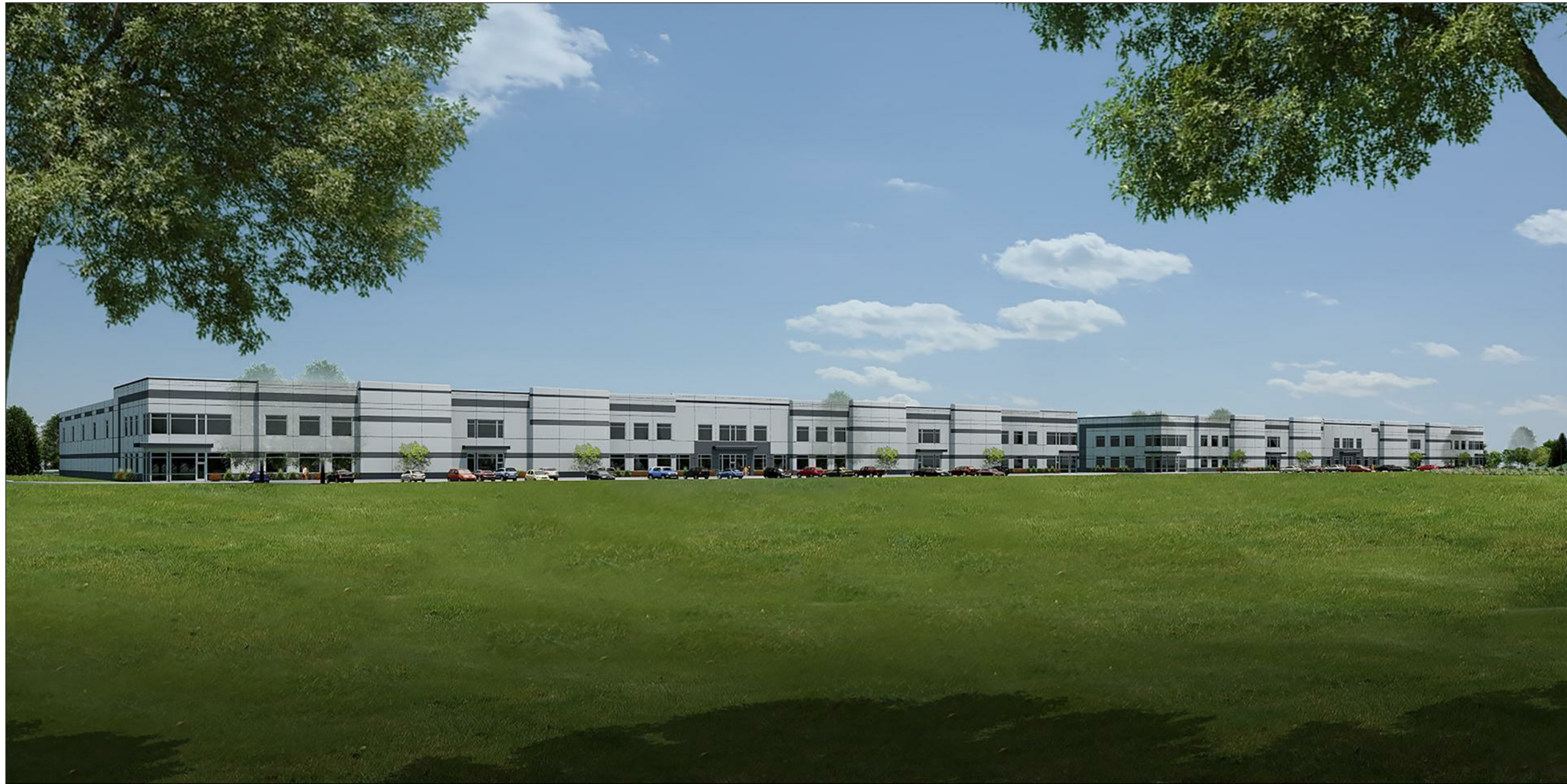
3 SOUTH WEST BUILDING - VIEW OF SOUTH WEST CORNER LOOKING NORTH / NORTH EAST NO SCALE
