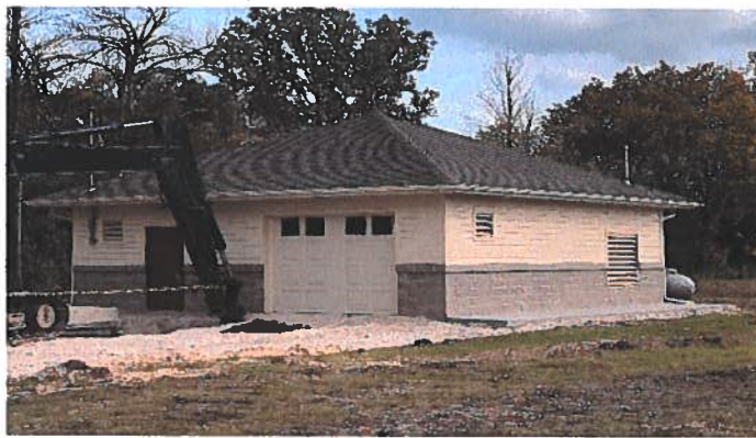
Wrenwood Sewage Pump Station
