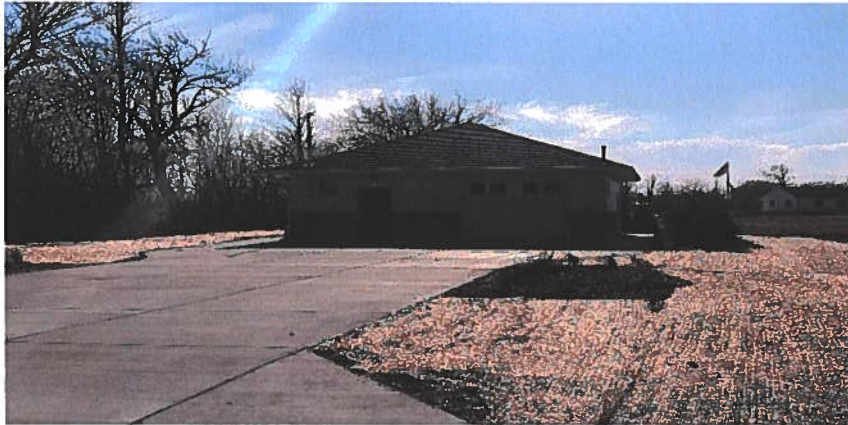
Wrenwood Sewage Pump Station_ Nov. 5, 2020
