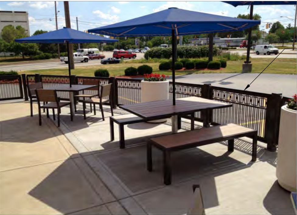
TACO BELL: NEW RAILING SYSTEM
