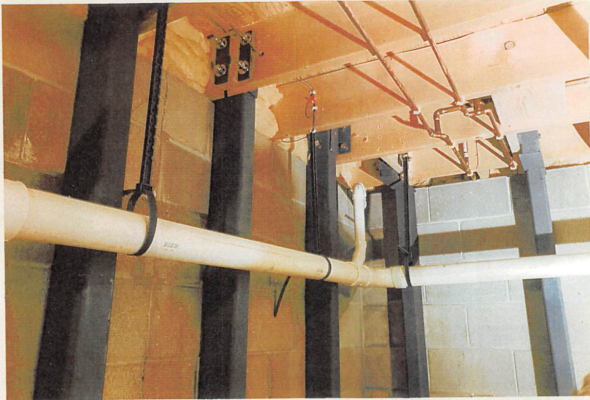
SOUTH EAST CORNER
