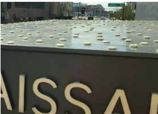
Optical Gel dishes placed strategically on this hotel's roof relocated a well entrenched flock of pigeons.
