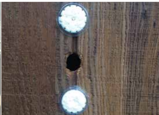
Dishes can be mounted vertically to protect wood structures against woodpeckers.
