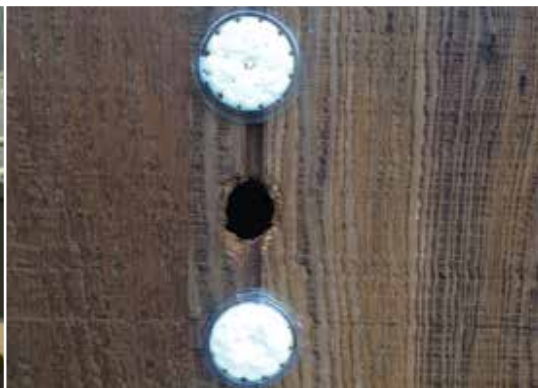
Dishes can be mounted vertically to protect wood structures against woodpeckers.
