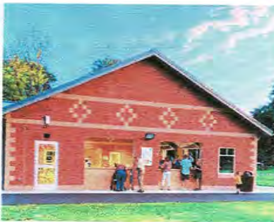
▲ Germantown Senior Center (above); Firemen's Park multi-use shelter (below)
