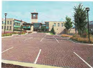
▲ Above photos show examples of permeable pavers in on-street and off-street applications
