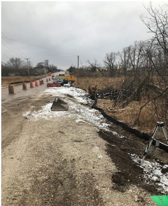
SANITARY SEWER INSTALLED ON DONGES BAY RD
