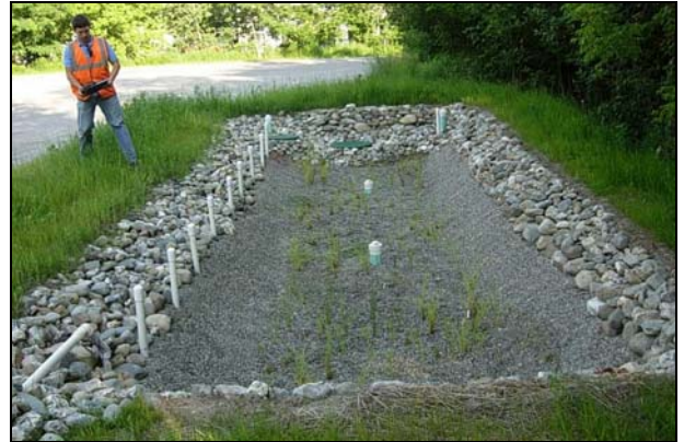
An example of a capital project construction (a gravel wetland) that was paid for by the stormwater utility in South Burlington, Vermont.
