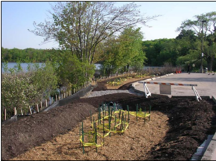
Two hydraulically connected bioretention cells paid for by the stormwater utility on Hammond Pond in Newton, Massachusetts
