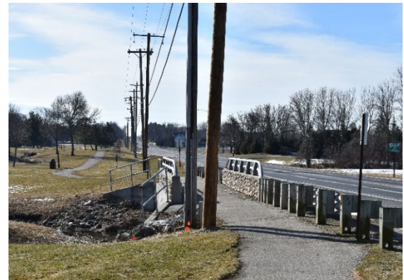
EXISTING PATH ON THE EAST SIDE
