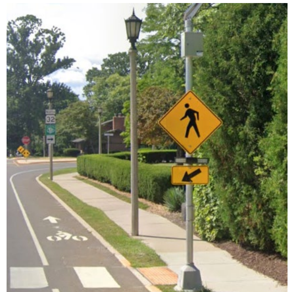
EXAMPLE OF AN ENHANCED CROSSWALK WITH HIGH VISIBILITY MARKINGS AND RRFB
