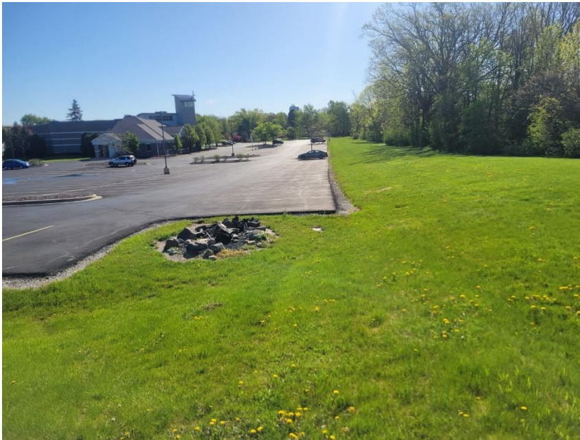
SW corner of parking lot looking east.
