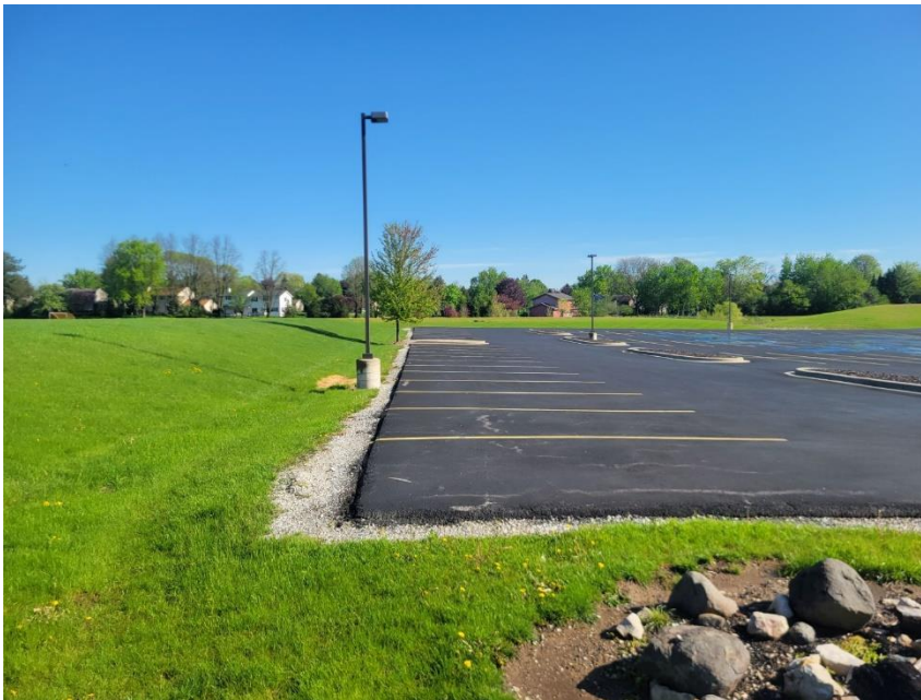
SW corner of parking lot looking north
