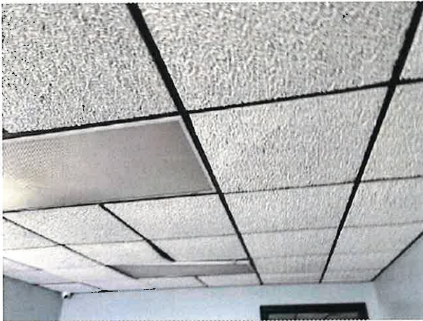
16. View of typical office ceiling building materials
