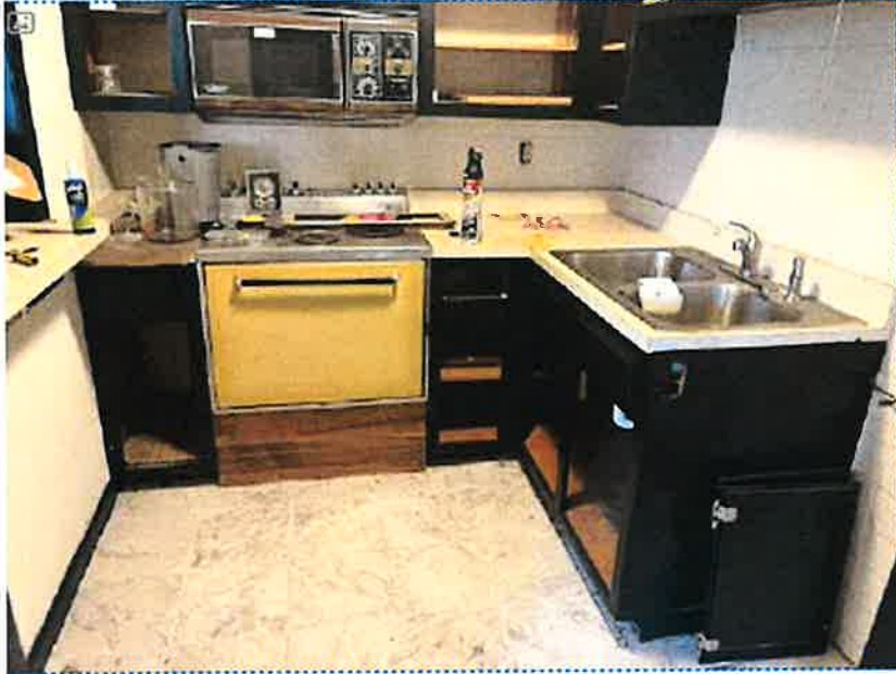
15. View of kitchen area
