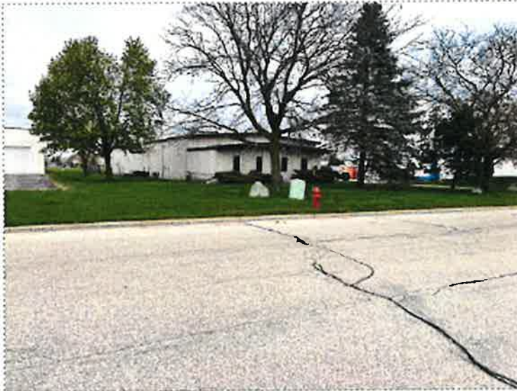
1. View of subject property facing northeast
