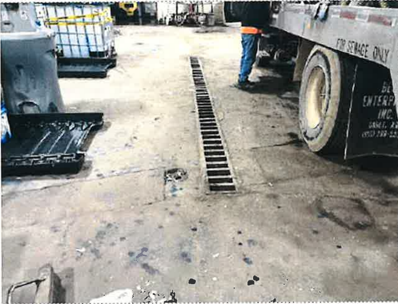
23. View of trench drain in warehouse area
