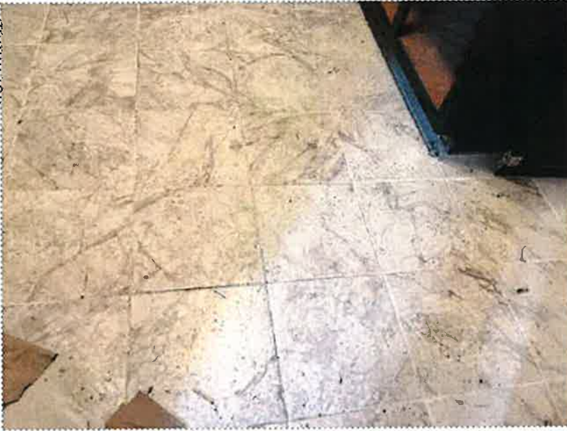
17. View of typical flooring surfacing material in kitchen
