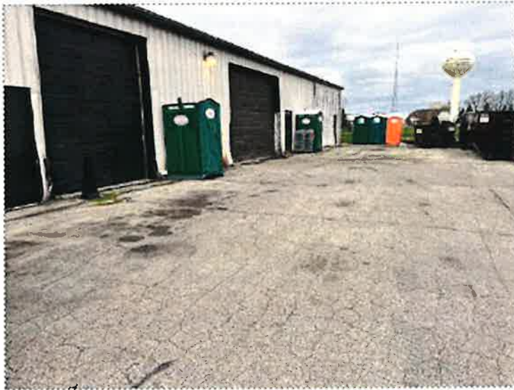
5. View of eastern elevation of subject property building
