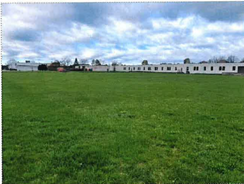
38. View of subject property - northern vacant parcel
