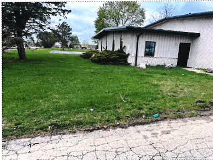
4. View of southern elevation of subject property building
