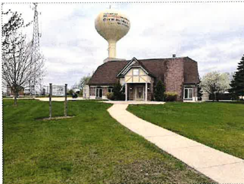
42. View of north adjoining property
