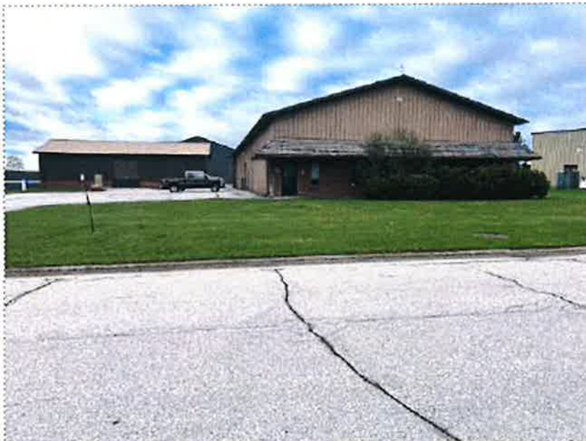
44. View of southwest adjoining property
