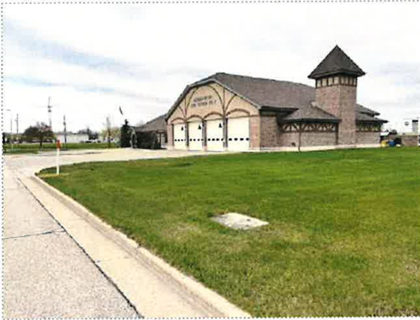
41. View of northwestern adjoining property
