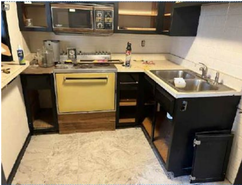
15. View of kitchen area
