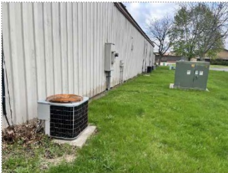
10. View of western elevation of subject property building
