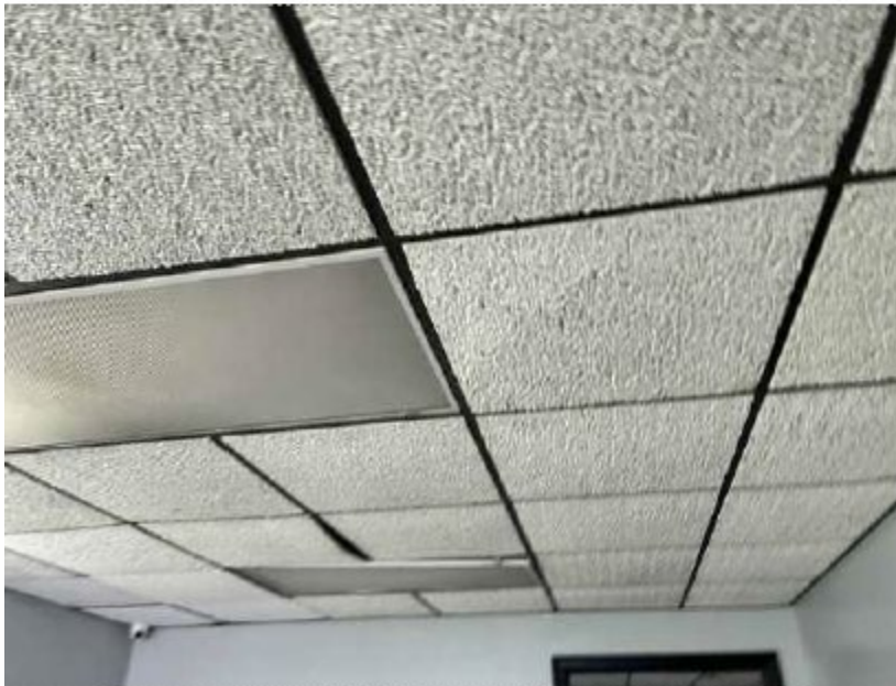
16. View of typical office ceiling building materials
