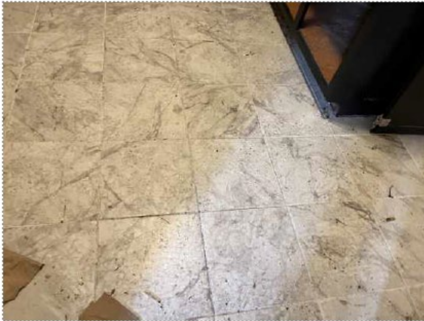
17. View of typical flooring surfacing material in kitchen
