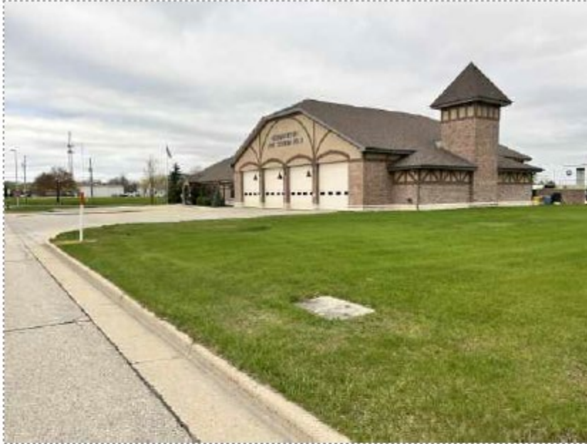
41. View of northwestern adjoining property
