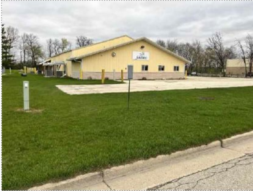
43. View of northeastern adjoining property
