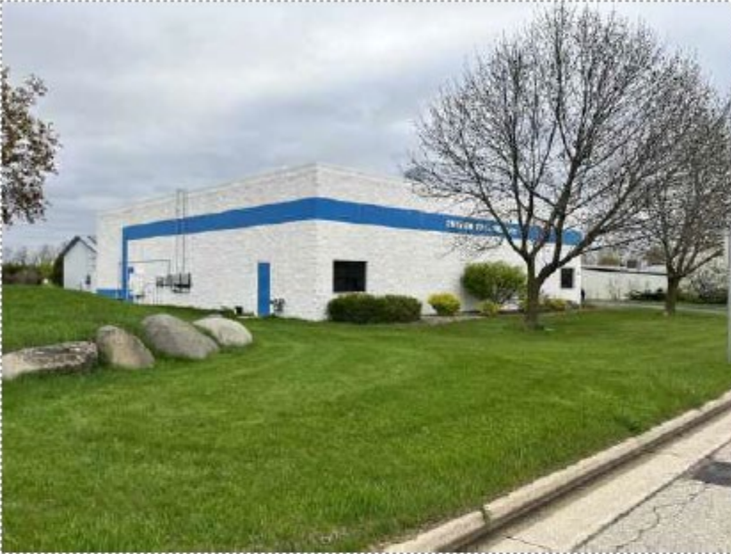
47. View of eastern adjoining property
