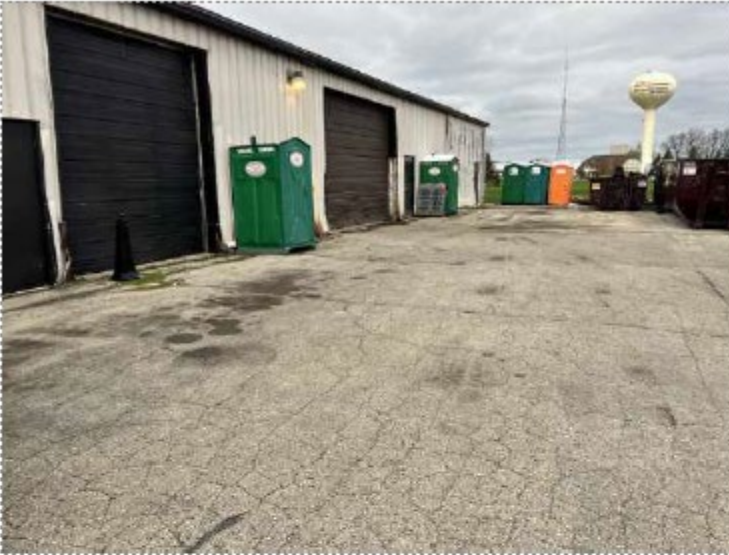
5. View of eastern elevation of subject property building
