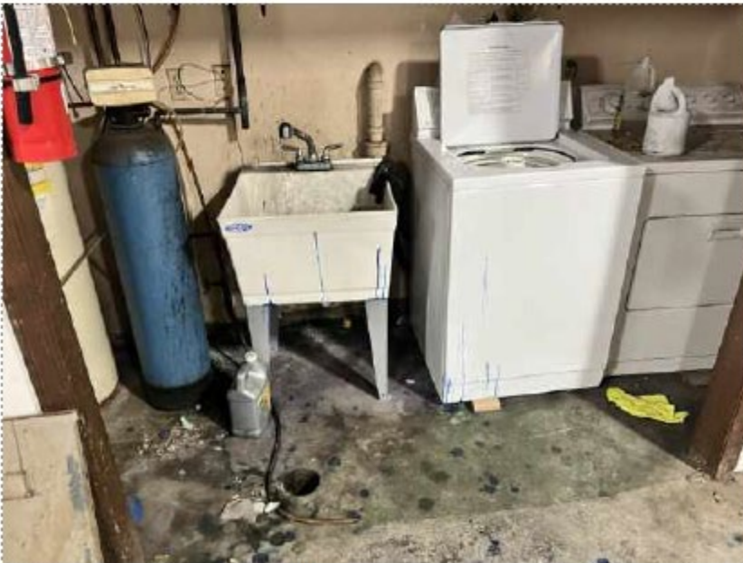
20. View of utility sink and janitorial closet
