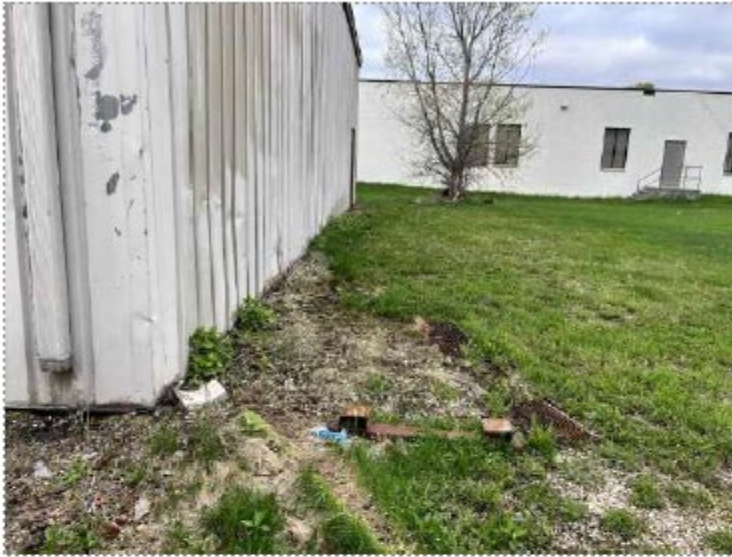
7. View of north side of subject property building:
