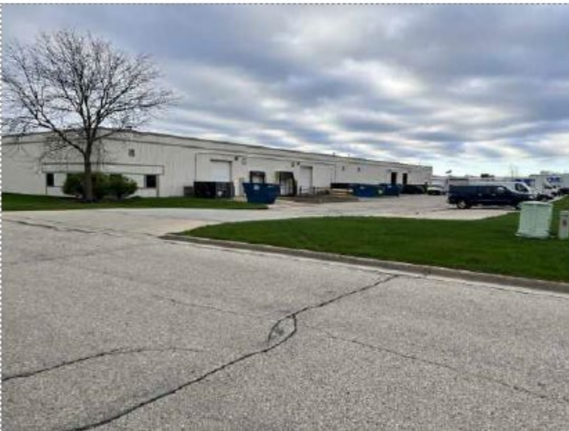
48. View of eastern adjoining property
