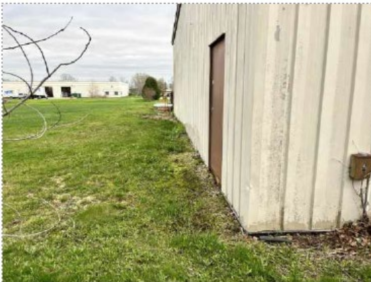
8. View of north side of subject property building:
