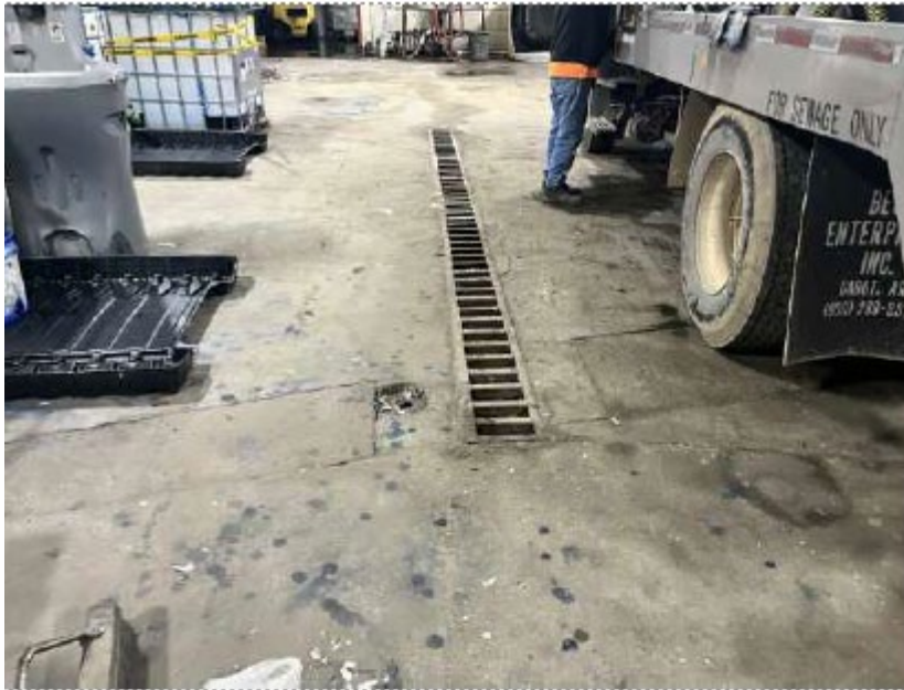
23. View of trench drain in warehouse area
