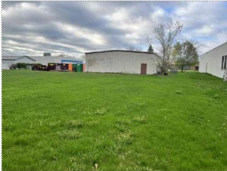
9. View of northern elevation of subject property building
