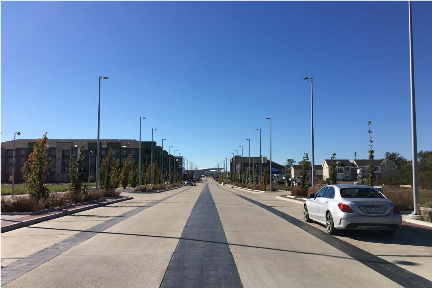
CHANGES IN PAVEMENT TYPE, CONTINUOUS ON-STREET PARKING, AND BUMP OUTS ENCOURAGE TRAFFIC TO SLOW AND PROVIDE PROTECTION FOR PEDESTRIANS.
