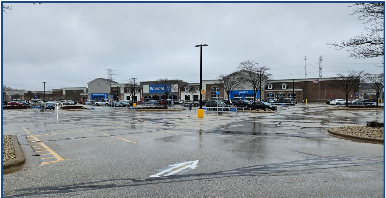
FRONT VIEW (FROM 2024 INSPECTION)
