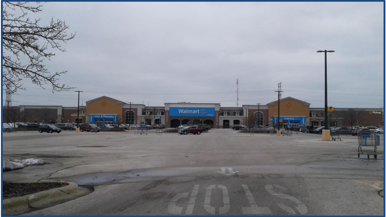
FRONT VIEW (FROM 2021 INSPECTION)
