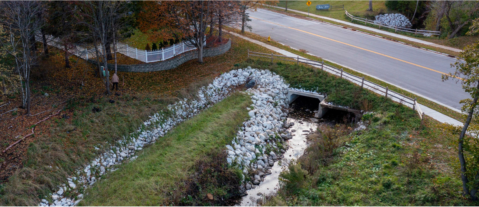
Waukesha Area 7 Stormwater Management - Waukesha, WI
