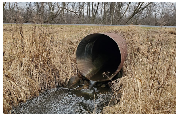
Before: Perched Culvert
