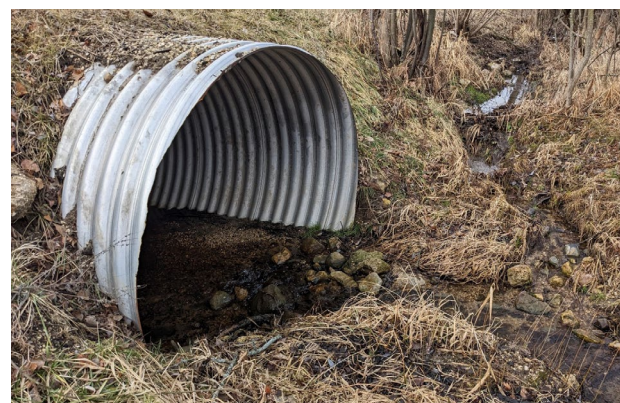
After: Perched Culvert
