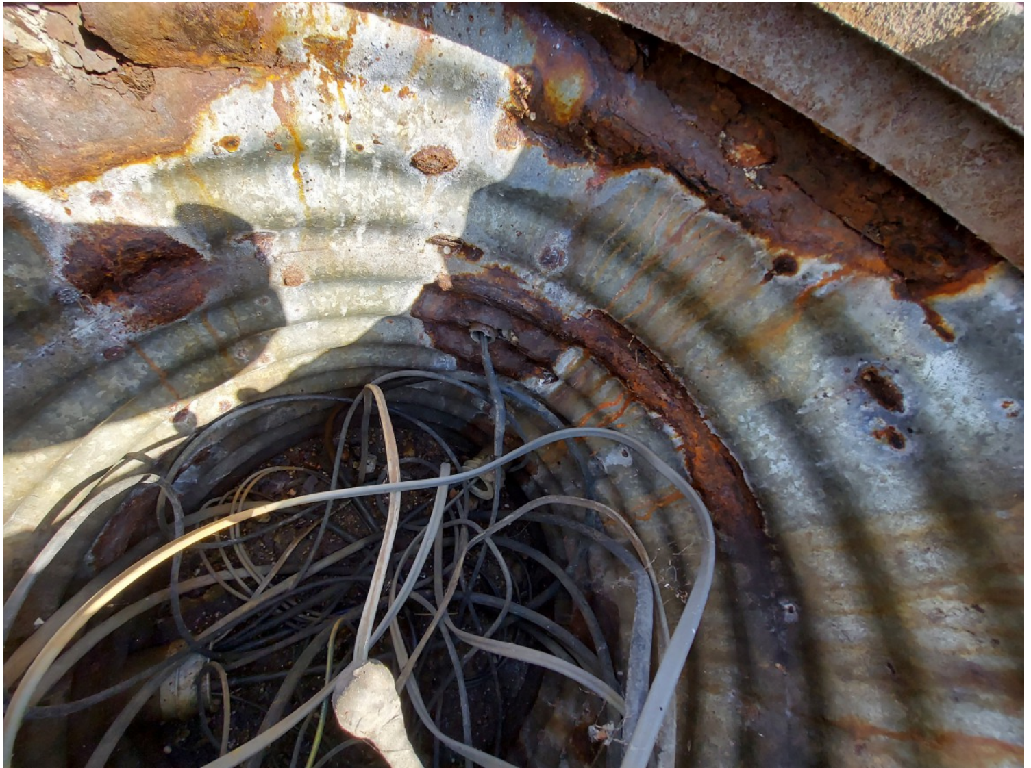
NW Island Manhole
