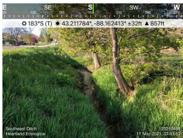
Photo #5 Photo of southeast ditch (WW-3)
