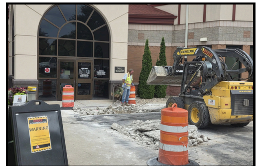
Construction to the library sidewalks has been going on since mid-July
