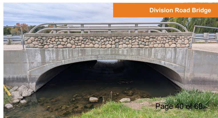
Maple Road Bridge
