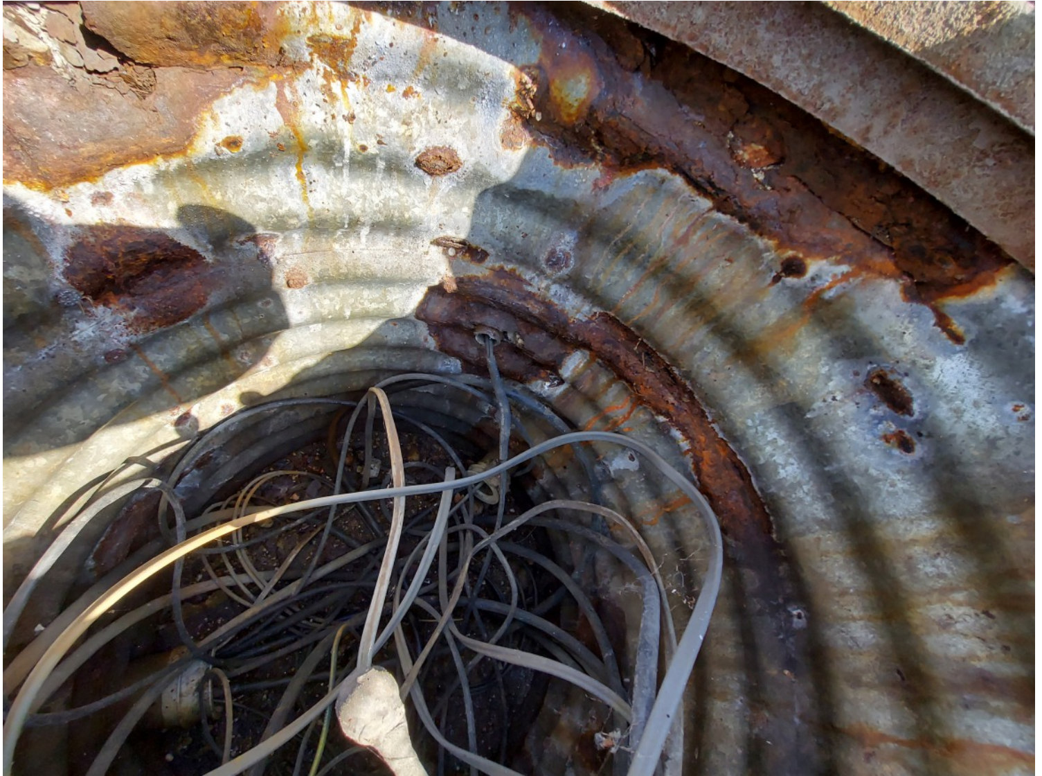
NW Island Manhole
