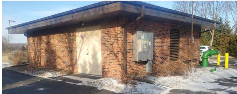
Old Farm Lift Station
