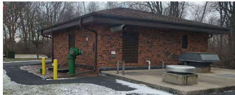
Main Street Lift Station
