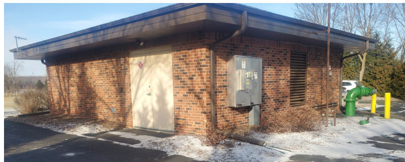
Old Farm Lift Station
