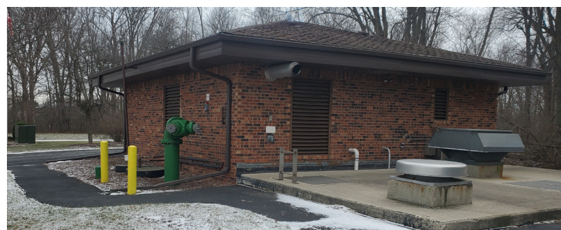
Main Street Lift Station
